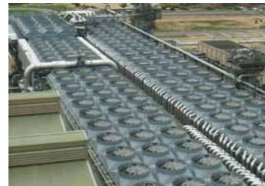
Air Fin Coolers (induced draft) Bonny Island, Nigeria
