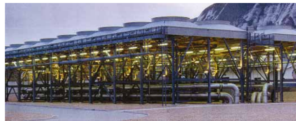
Air Fin Coolers (induced draft) Chillers for Eurotunnel, England/France
