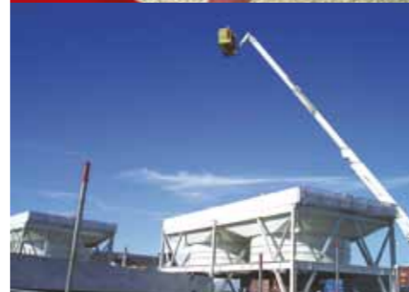
AFC and ACC testing Shop run-in tests may include vibration, air flow, power consumption and noise level measurement.
